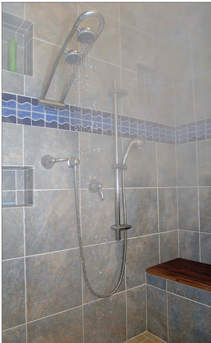
Wheelchair accessible shower built by Legal Eagle Contracting.
